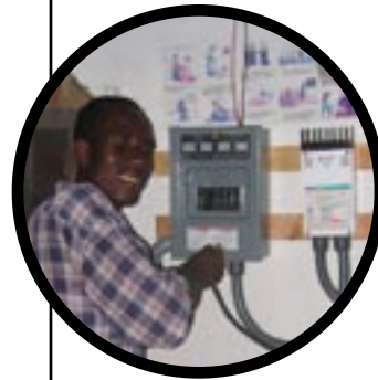
The installation of charge controller and circuit breaker box in a PV system
