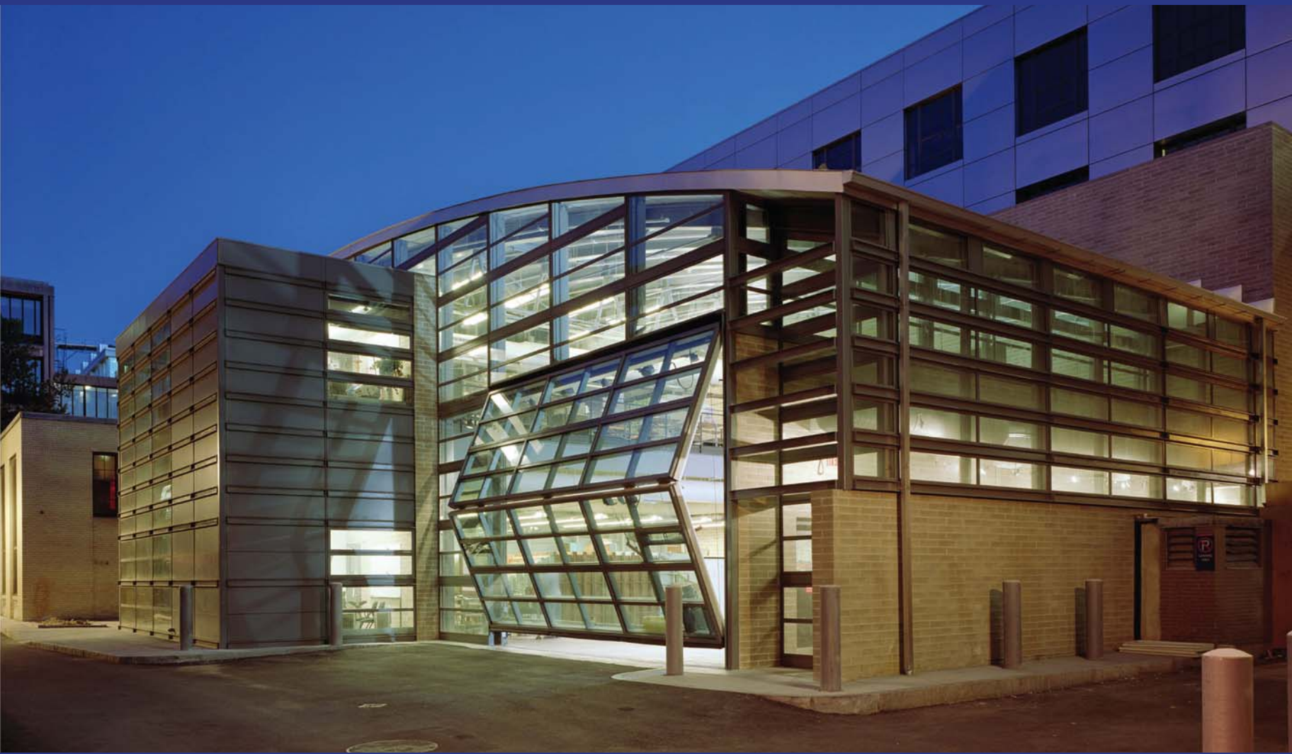
The Gerhard Neumann Hangar, added to the rear of Building 33 as part of the MIT Department of Aeronautics and Astronautics Learning Laboratory, offers space for students to construct and test large projects. See article, page 15. (Nick Wheeler photograph, Cambridge Seven Assoc.)
