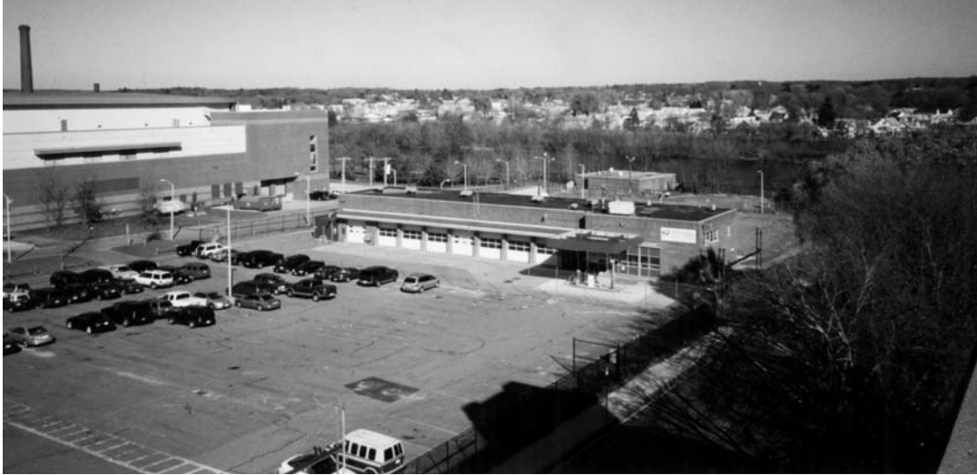
The existing postal facility (center) is ideally situated on the banks of the Merrimack River and adjacent to the Tsongas Arena (shown to the left).
