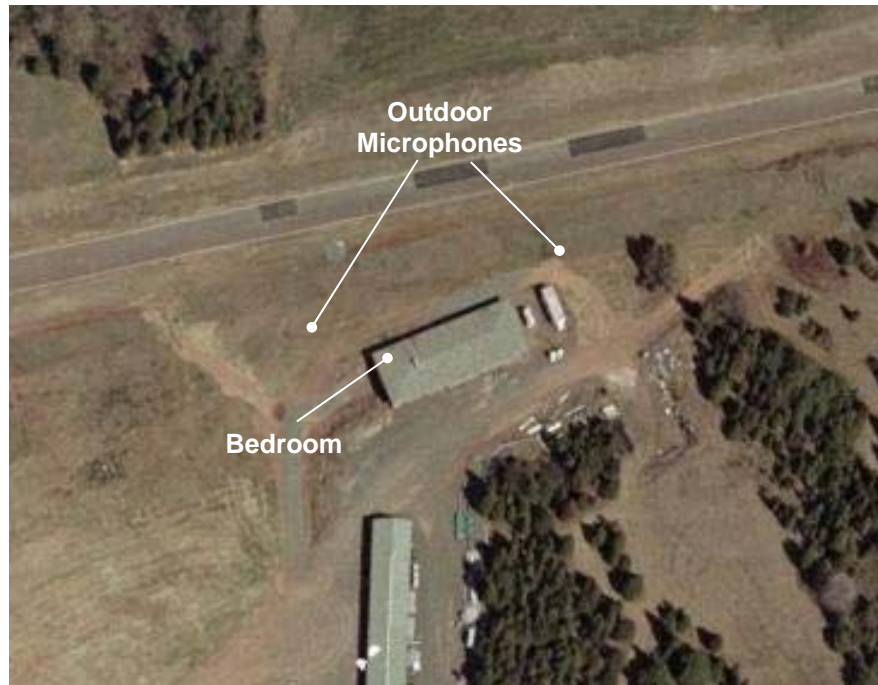
Figure 9. Overhead photograph of the Stone House indicating the instrumented bedroom and approximate location of the two outdoor microphones. Runway 1R is approximately 2700 ft (820 m) to the right, Runway 30 is 3100 ft (960 m) to the left. North is up in this photograph. (The two small structures that appear in this image to the right of the Stone House were not present during the field study.) (Image courtesy of the USGS.)
