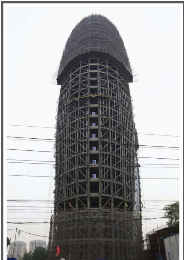
An investment to last a thousand years? In the shocking future of MIT 2031, the new Grimson Administrative Building dominates the campus.
